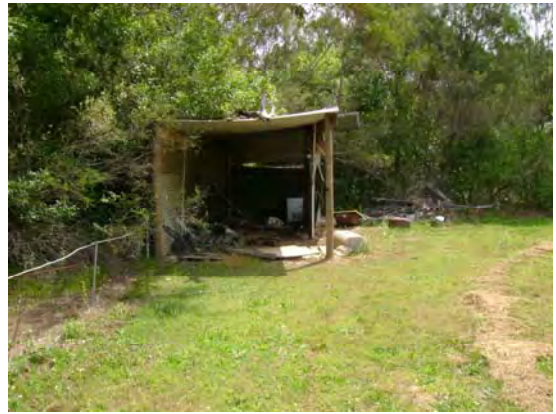
Figure 4: Old shed on cleared paddock
